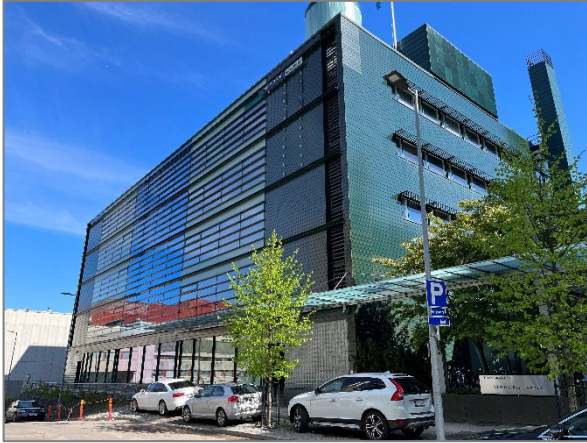
Facade to Televisiokatu
