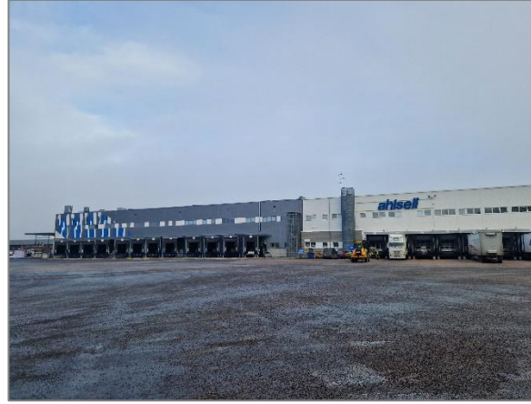
Front yard and facade, loading area
