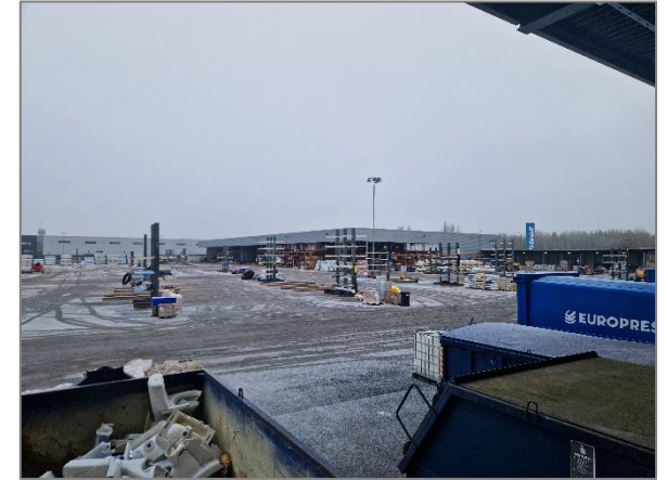
Seperate open warehouse shelter / building
