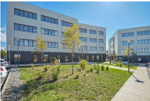
Exterior view of the “Beehive” complex, ©Swiss Life Asset Managers France
