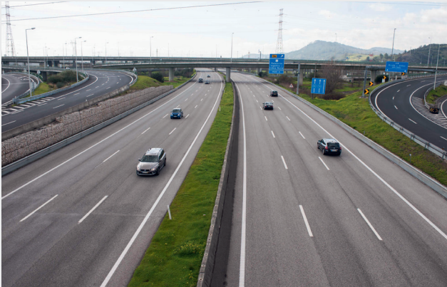
Section of the A1 motorway connecting the main Lisbon-Porto axis. Source: Brisa
