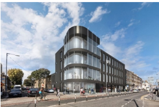
47-51 Richmond Street South, Dublin
