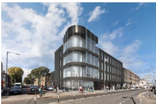
47-51 Richmond Street South, Dublin
