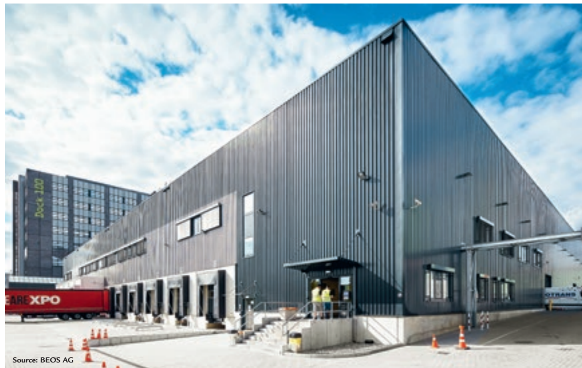
In the "Dock100", BEOS AG developed a distribution centre of around 13,700 square metres from which Berlin's inner city districts are serviced within an hour.
