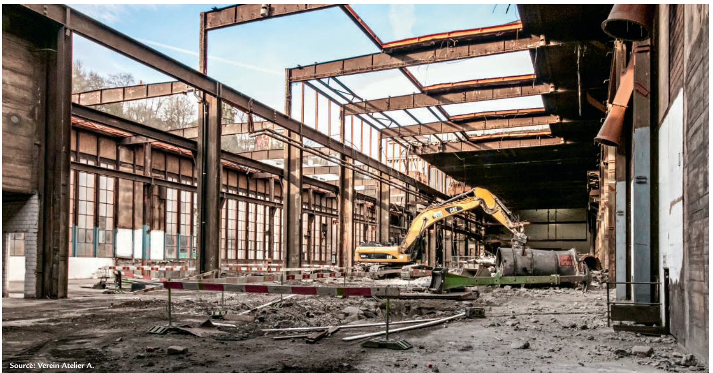
A new urban district takes shape on the site of an old steelworks.
