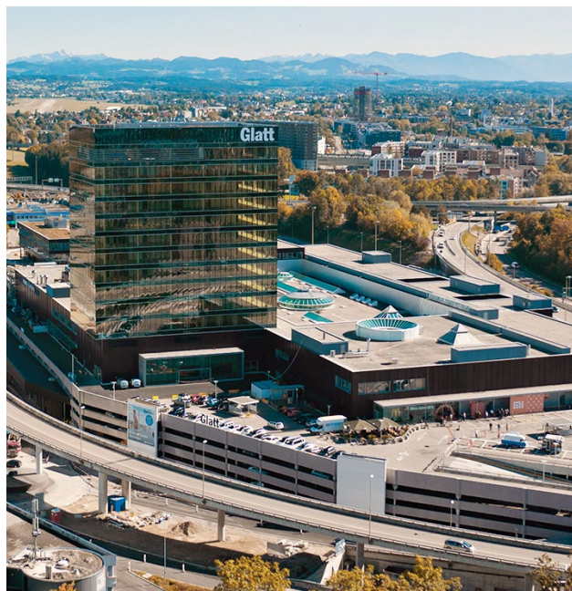
The Glatt centre is one of Switzerland's most successful shopping centres.
